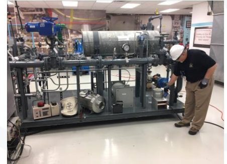
Plant mock-up – instructor hiding TWR source
